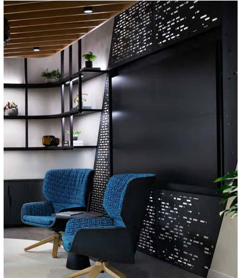
Laser cut steel panels in custom pattern + steel tube shelving Prevolve
