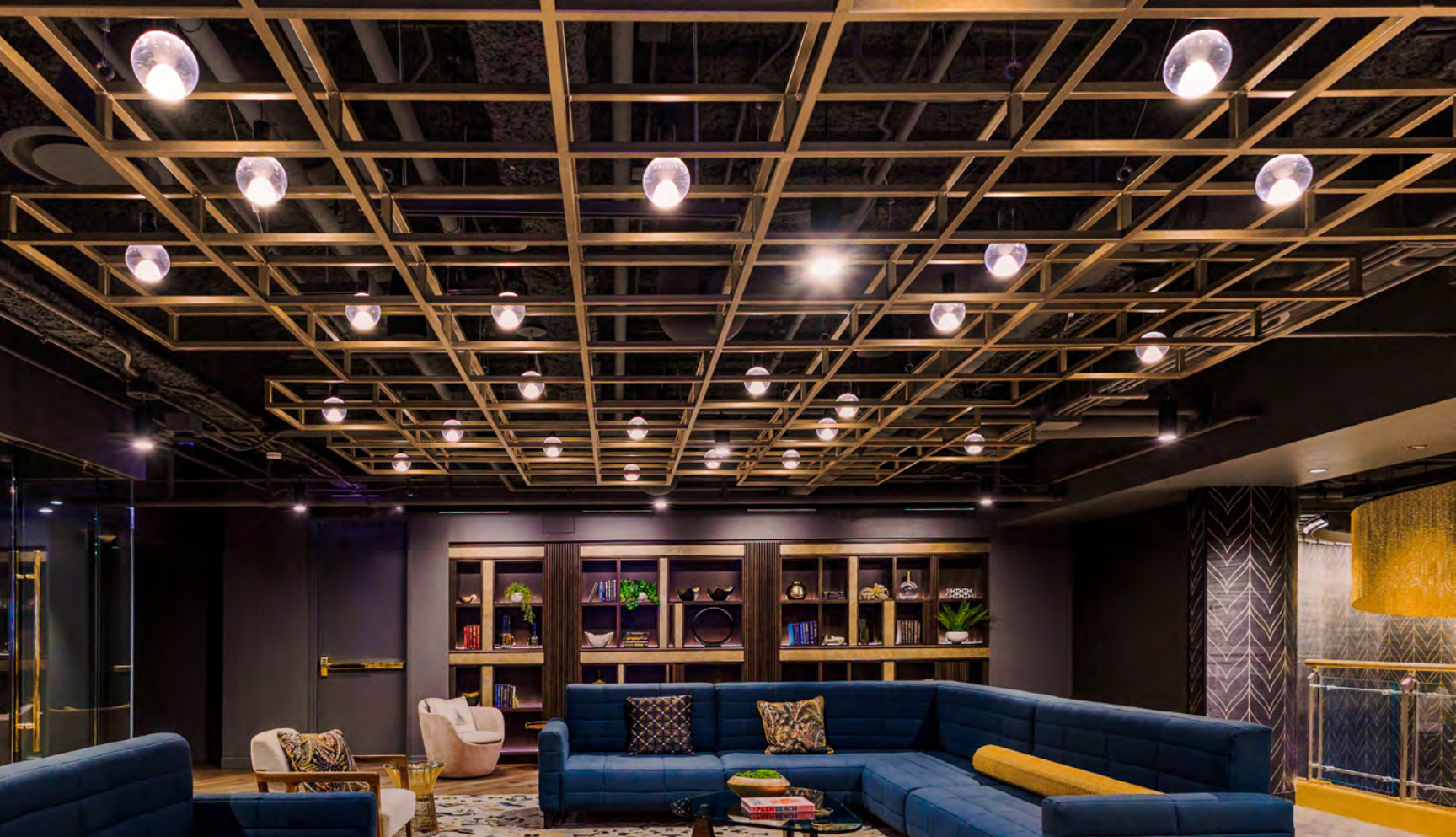
Steel tube grid ceiling element in custom shape + brass color powdercoat Wright Hereema Architects
