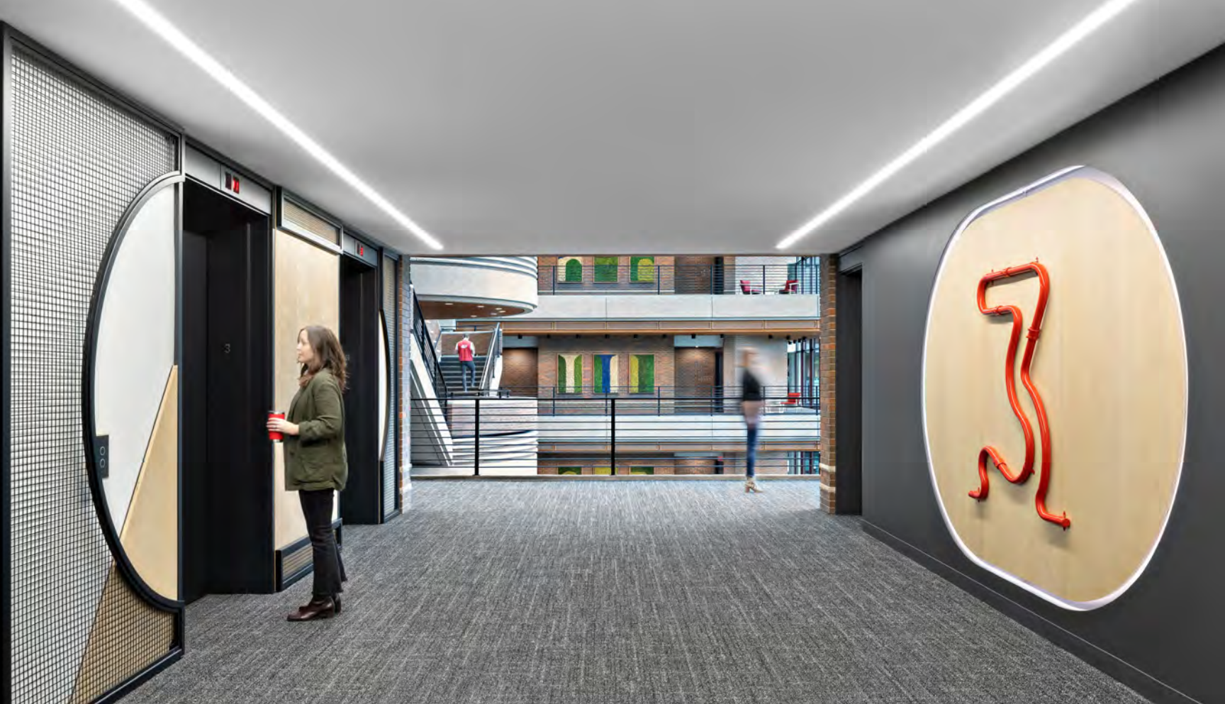
Left: Arched steel tube + wire mesh infill | Right: Bent steel pipe elevator signage + red color powdercoat CBRE Design Collective
