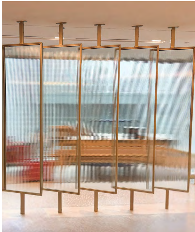
Steel tube frame + reeded glass infill + custom color powdercoat Lamar Johnson Collaborative
