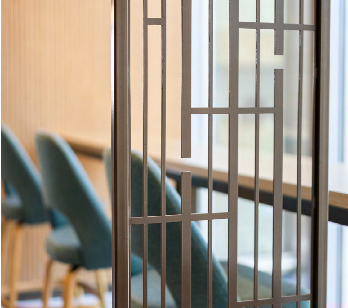
Laser-cut steel space divider in custom pattern + custom color powdercoat SmithGroup
