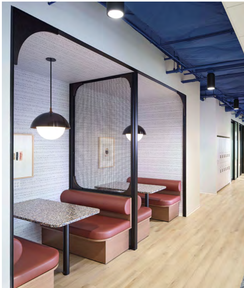
Steel tube frame + wire mesh infill + wood trim booth divider CBRE Design Collective
