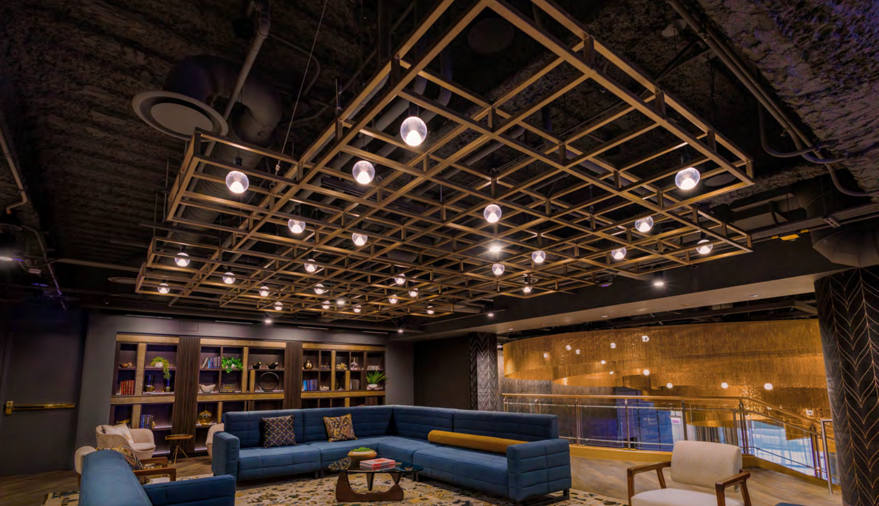
Steel tube grid frame in custom shape + custom color powdercoat Wright Hereema Architects
