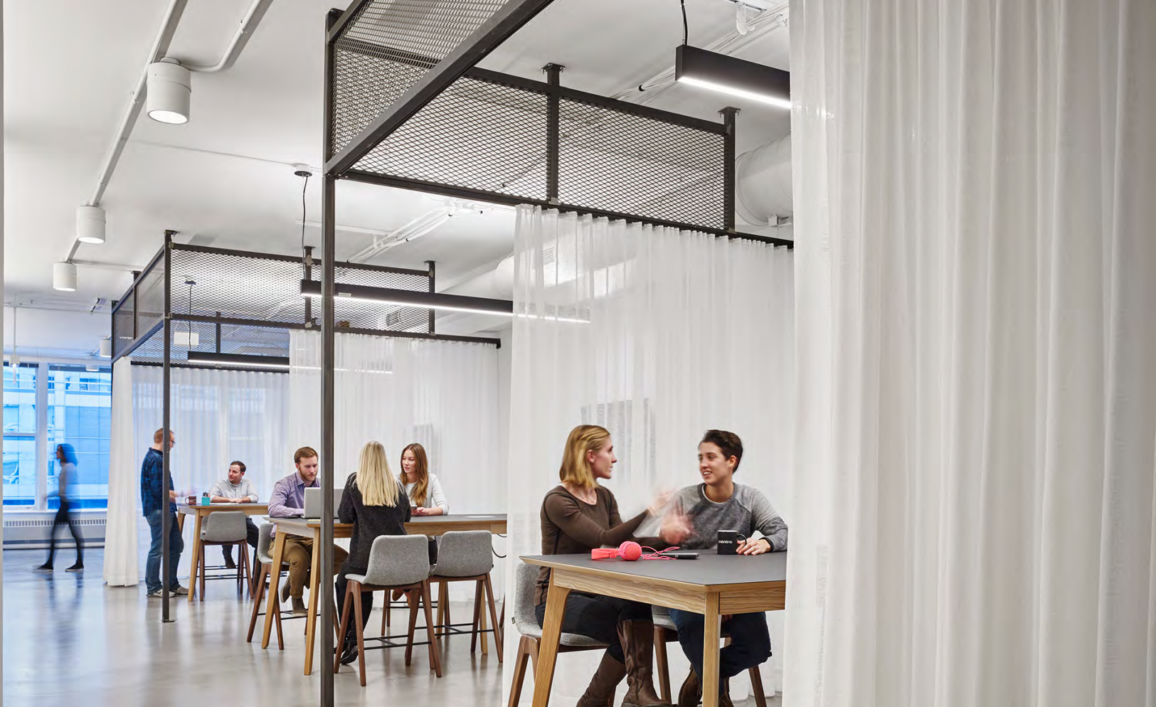
Steel tube canopy frame + expanded metal infill + curtains Partners by Design
