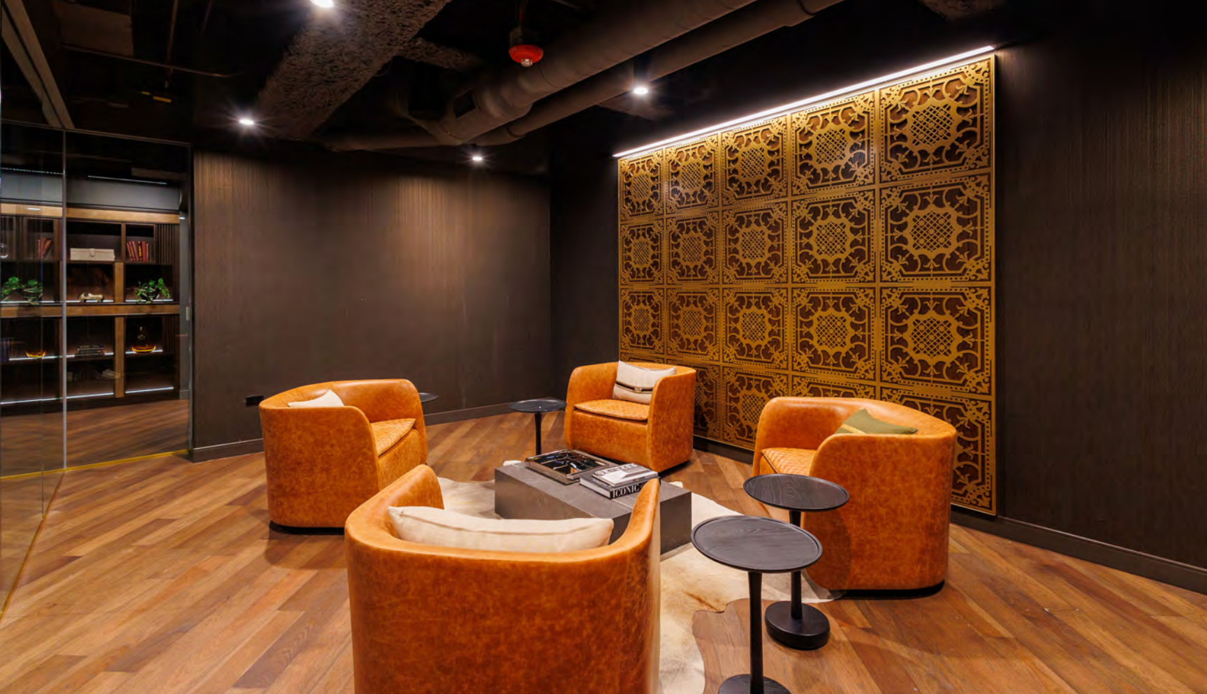
Feature wall: steel water-jet patterned design + custom color powdercoat + walnut veneer back paneling Wright Hereema Architects
