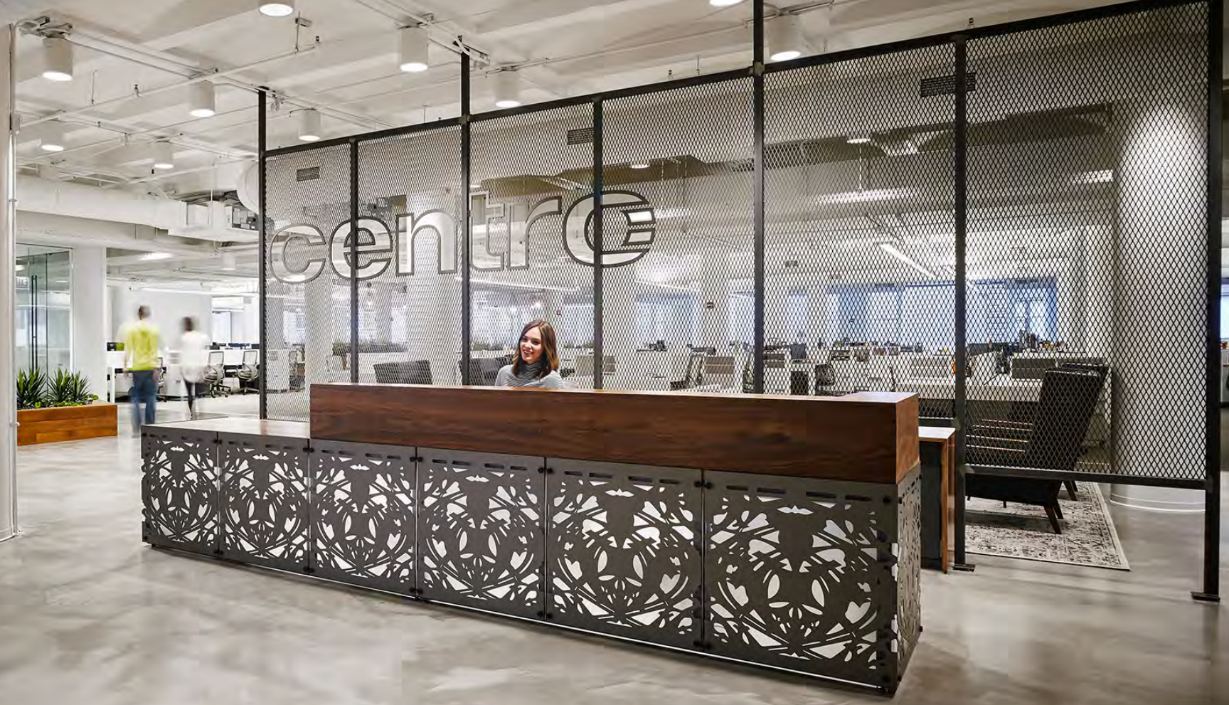
Steel space divider + laser-cut custom logo | Steel plate reception desk face + custom laser-cut pattern Partners by Design
